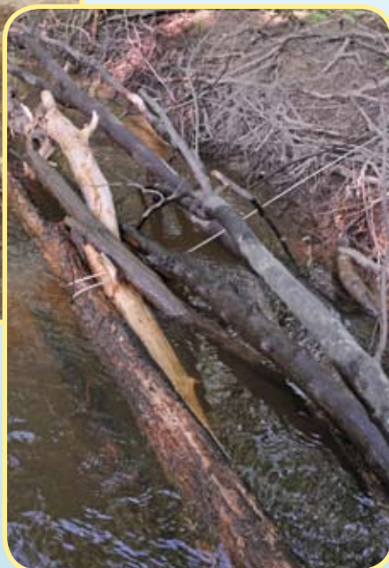
Figure 56 - Logs cabled together to armor eroding bank
