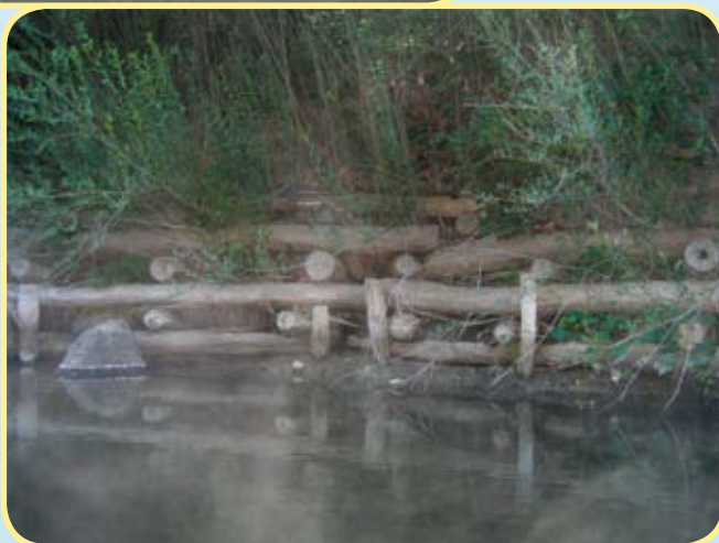
Figure 48 - Log matrix used to armor bank
