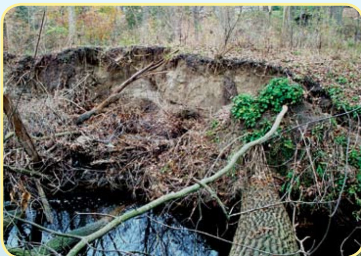
Figure 59 - LWD structure causing bank erosion
