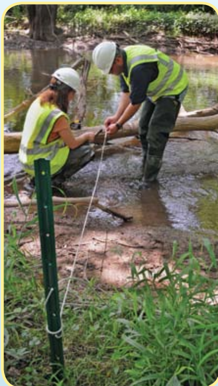
Figure 50 - Anchoring a log using the Palmiter Method
