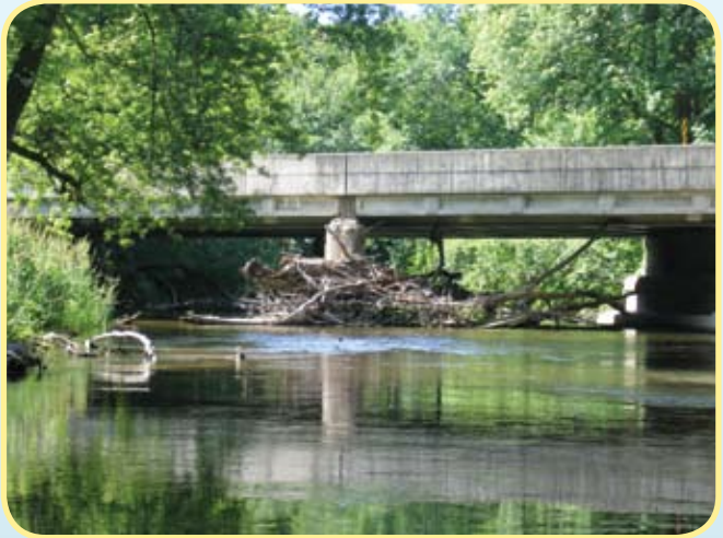
Figure 42 - LWD blocking culvert
