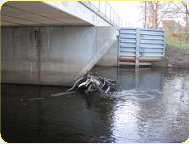
Figure 40 - Minor LWD accumulation on bridge pier
