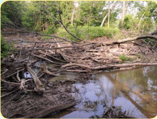
Figure 37 - An anchored debris dam
