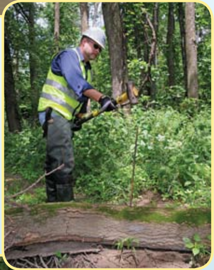
Figure 32 - Anchoring log to bank with rebar
