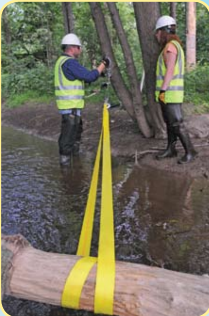
Figure 29 - Using a come-along to reposition log
