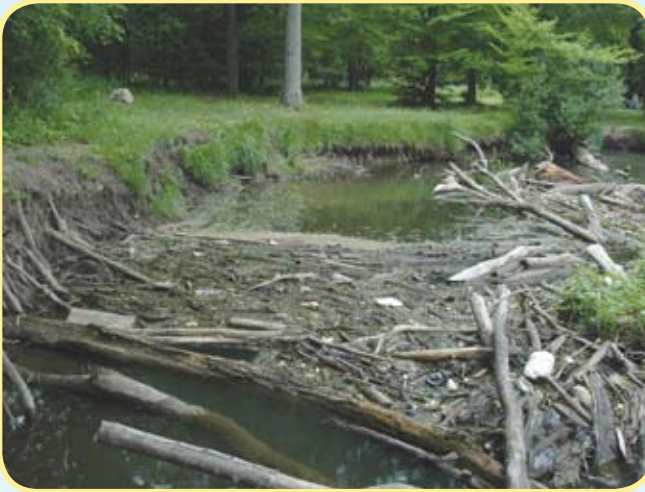
Figure 34 - A floating debris dam
