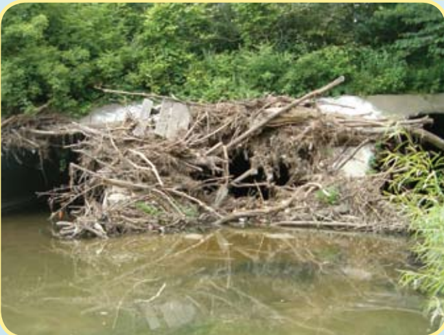
Figure 42 - LWD blocking culvert
